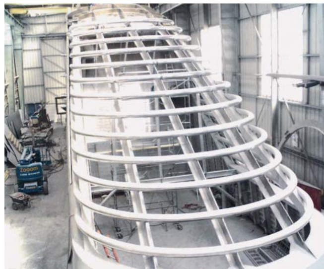
Ship's funnel under construction
