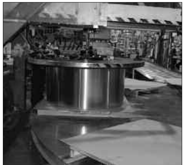
Figure 15 - Moving Coils with a Vacuum Lift
