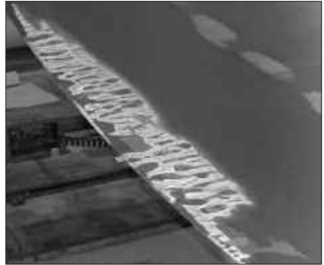
Figure 1B - Water Stain on Sheet
